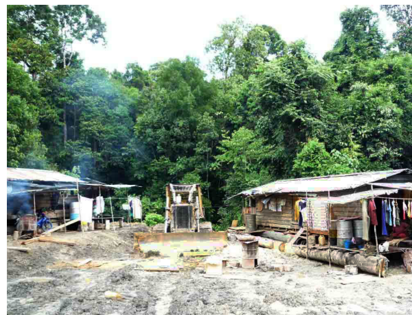
A shack in a logging camp at Anap-Muput: the shack is built on huge logs. A bulldozer is used to shift it along as camp sites move to other areas.
