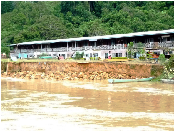
Photo4: Riverbank erosion in slip-off slopes (Type II) According to the residents the riverbank collapsed during the period of flood when express boat generated waves hit the bank.
