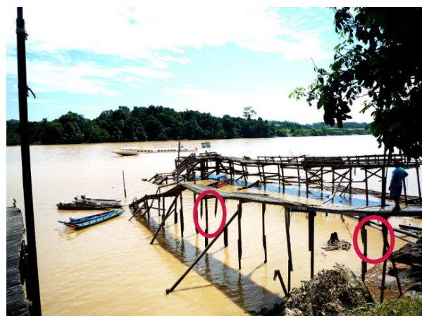
Photo7: Old short stakes can be seen on the frame of boarding bridge In this photo, shorter stakes can be seen in encircled areas. Those stakes were in use before as the slope of the riverbank was far gentler but because of the erosion the slope of the bank became much lower than before. The interview with the residents confirmed the fact.
