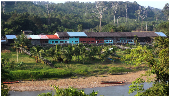
Photo 2: An Iban longhouse located in the most upstream area of the Anap River
