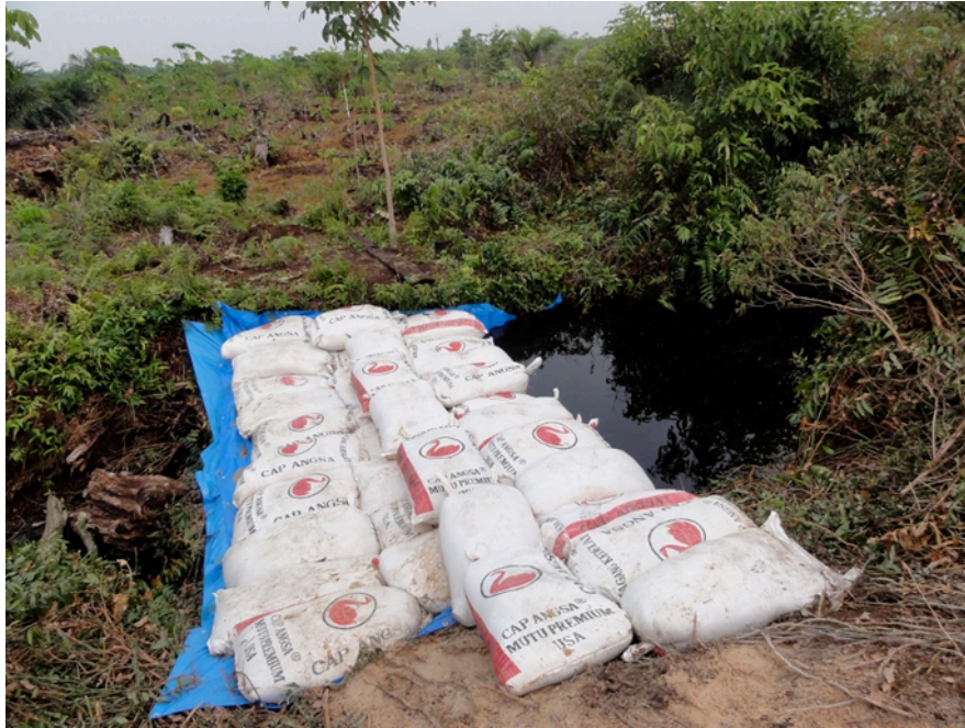
Fig. 1 Simple dam constructed at the experimental site
