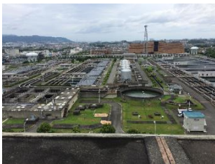
Murano water treatment plant
