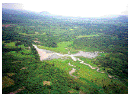
An old thamnop (traditional earthen weir) in Siemriap, Cambodia
