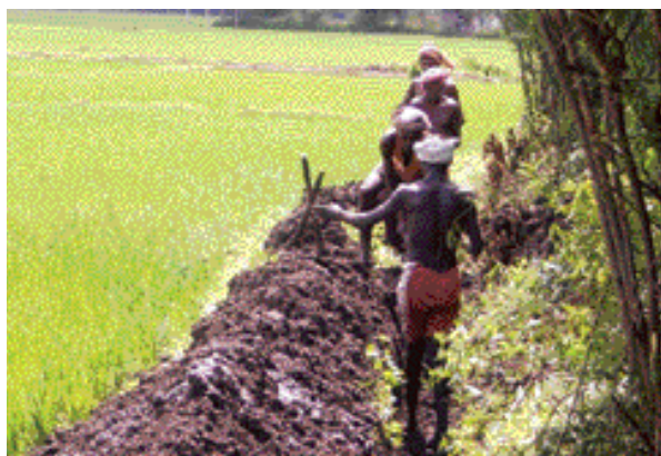
Tank maintenance work by command area farmers
