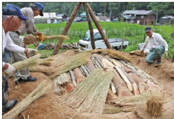
炭焼き窯づくり (滋賀県余呉町) Making Charcoal kiln (Yogo town, Shiga prefecture)
