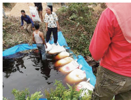
Simple dam for rewetting and preventing peat fires in a drainage canal, constructed by our FS and the local community
