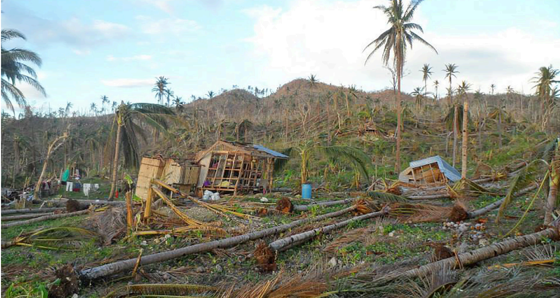
Fig. 2 Damages caused by super typhoon Haiyan in our village. It destroyed our houses and coconut trees.
