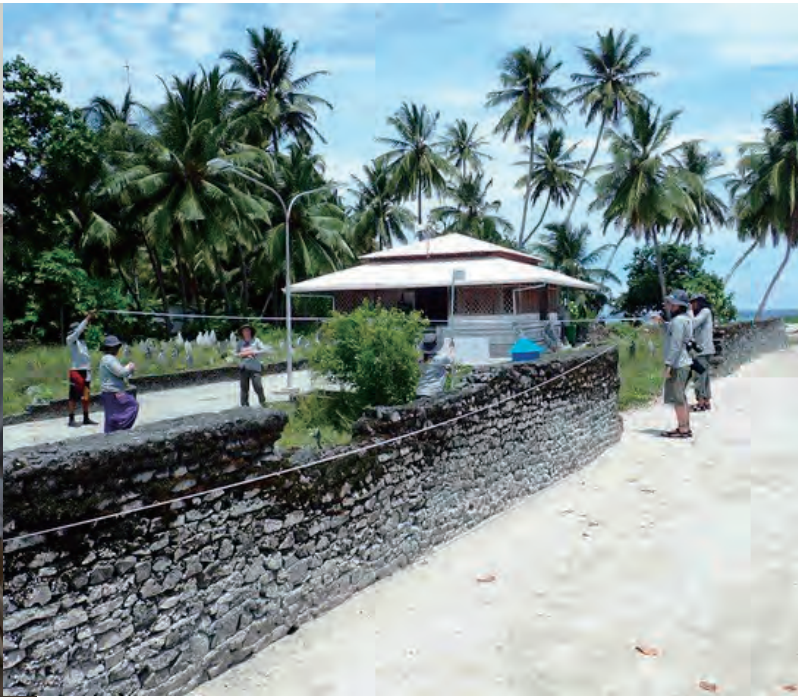
Work on site of a coral-stone mosque in Laamu Atoll
