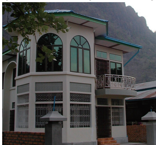
Fig. 2 A migrant-laborer’s house under construction
