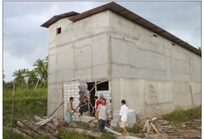
Building Swiftlet farmhouse in Sarawak, Malaysia.
